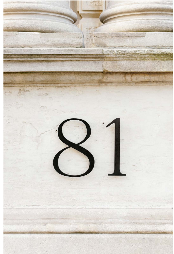
Both page: Grade-II Listed Masonry Facade 81 Colmore Row lies behind a stunning masonry facade with outstanding details
