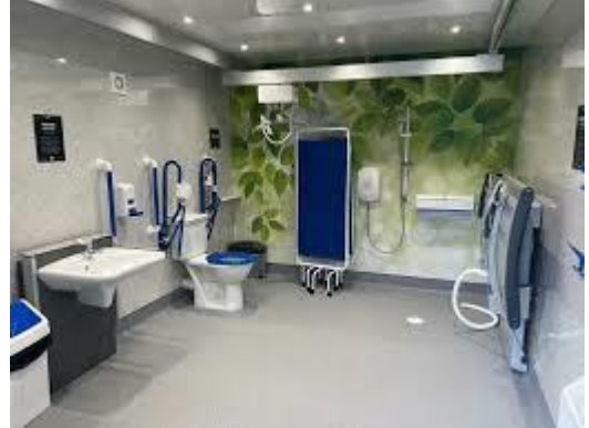
Changing Places Toilet
